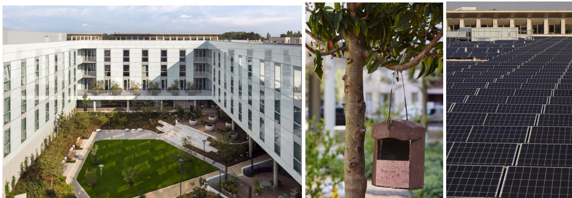
Turing Locke courtyard, bat boxes and solar panels.
